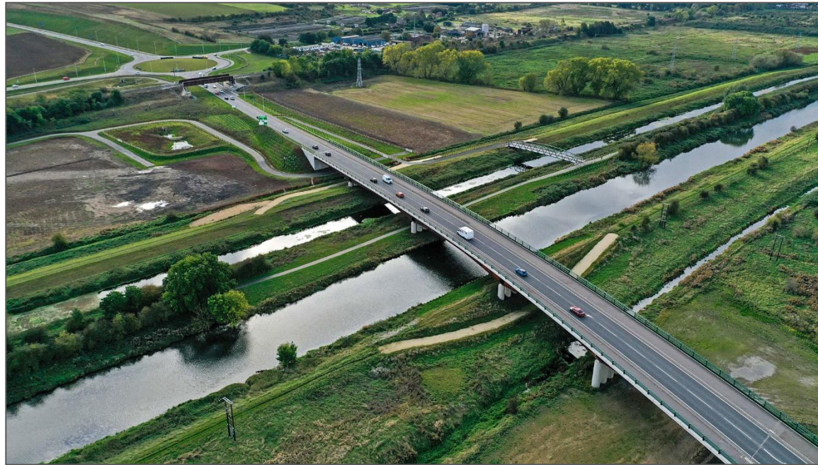
Figure 3 : Viaduct carrying the A15 Lincoln Eastern Bypass over the River Witham, after completion
