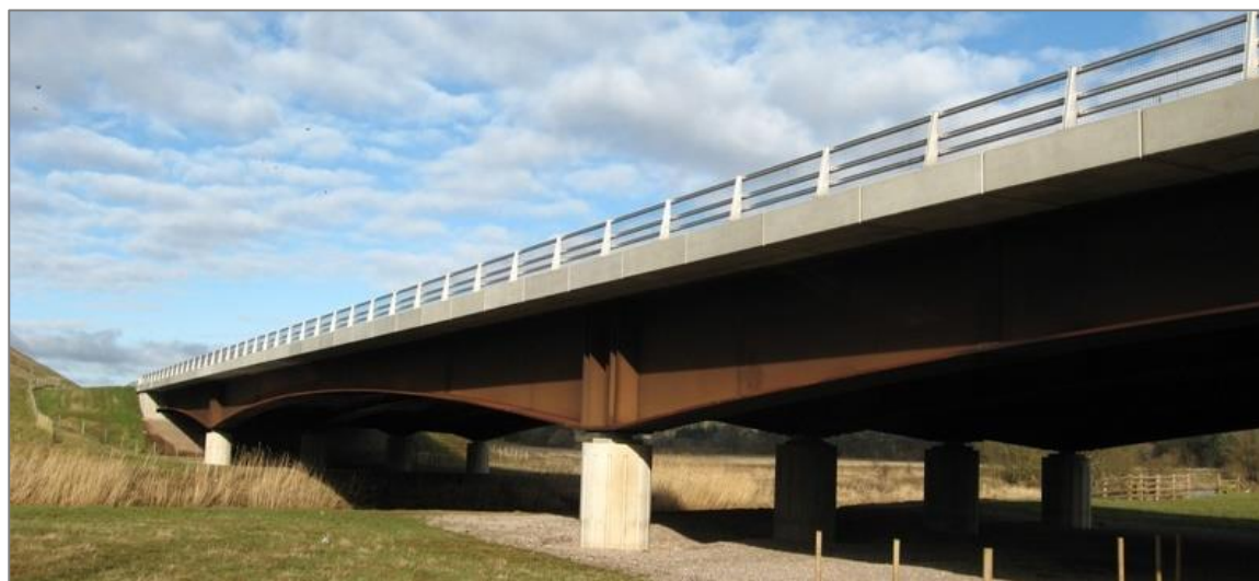
Figure 6: Example of a low-lying viaduct – River Eden Bridge
