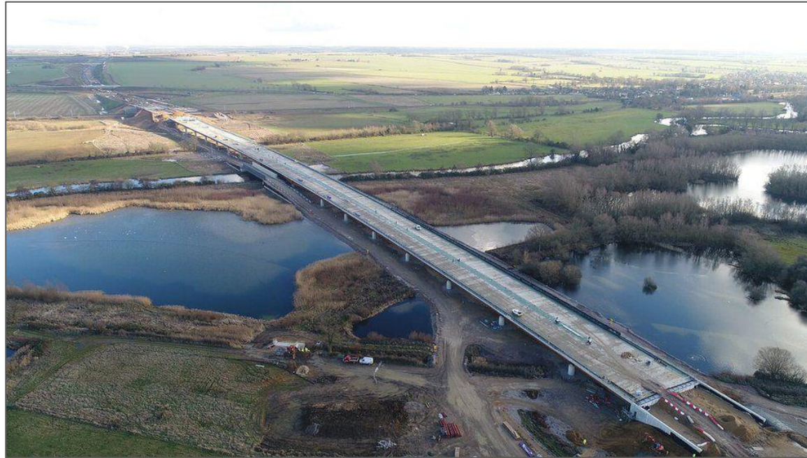
Figure 2 : Viaduct carrying the A14 over the River Great Ouse, under construction
